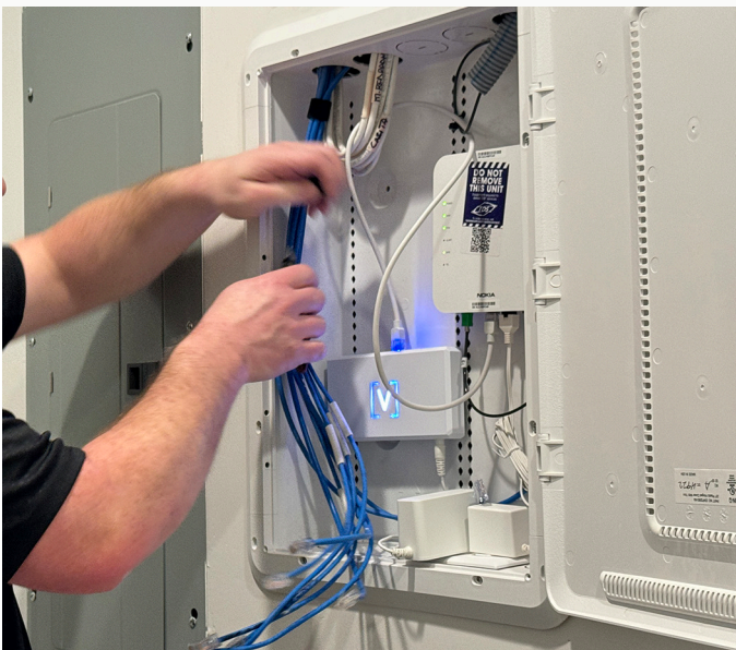
Installing the Alta Labs S8-POE Switch
